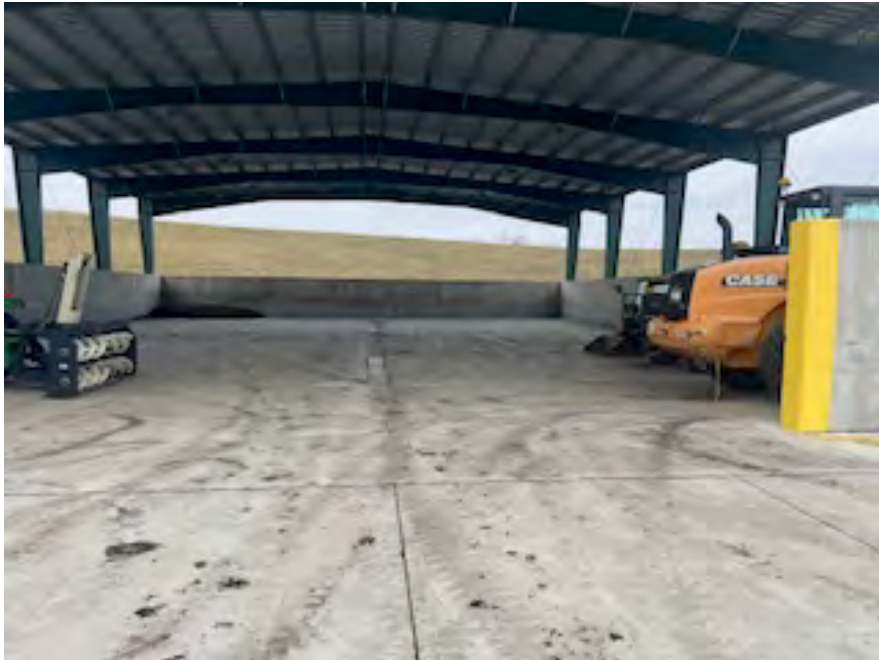
Biosolids Storage Bld. Empty and Washed Down
