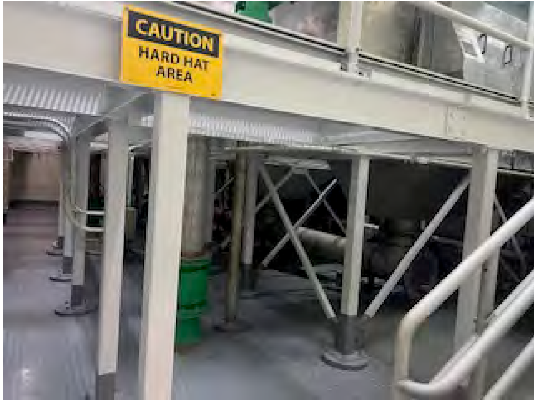
Fine Screen Room I Beams Repainted
