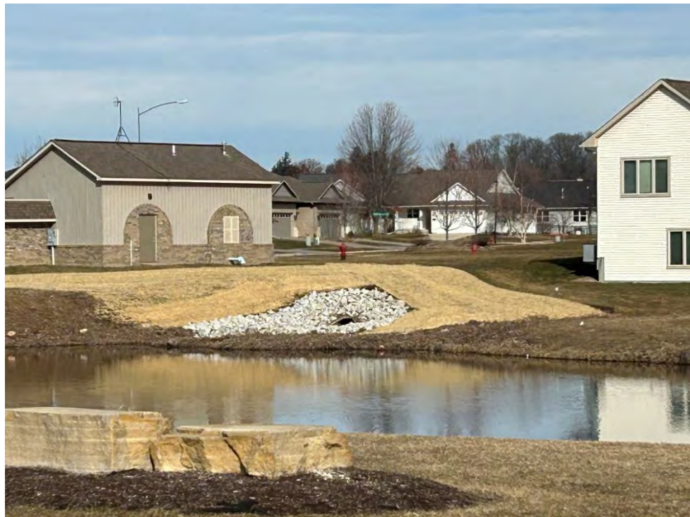
Cedar Springs outfall after
