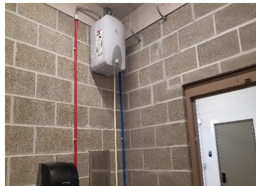
New sink and hot water heater installed at the Rec Center maintenance building (Old bike shelter).
