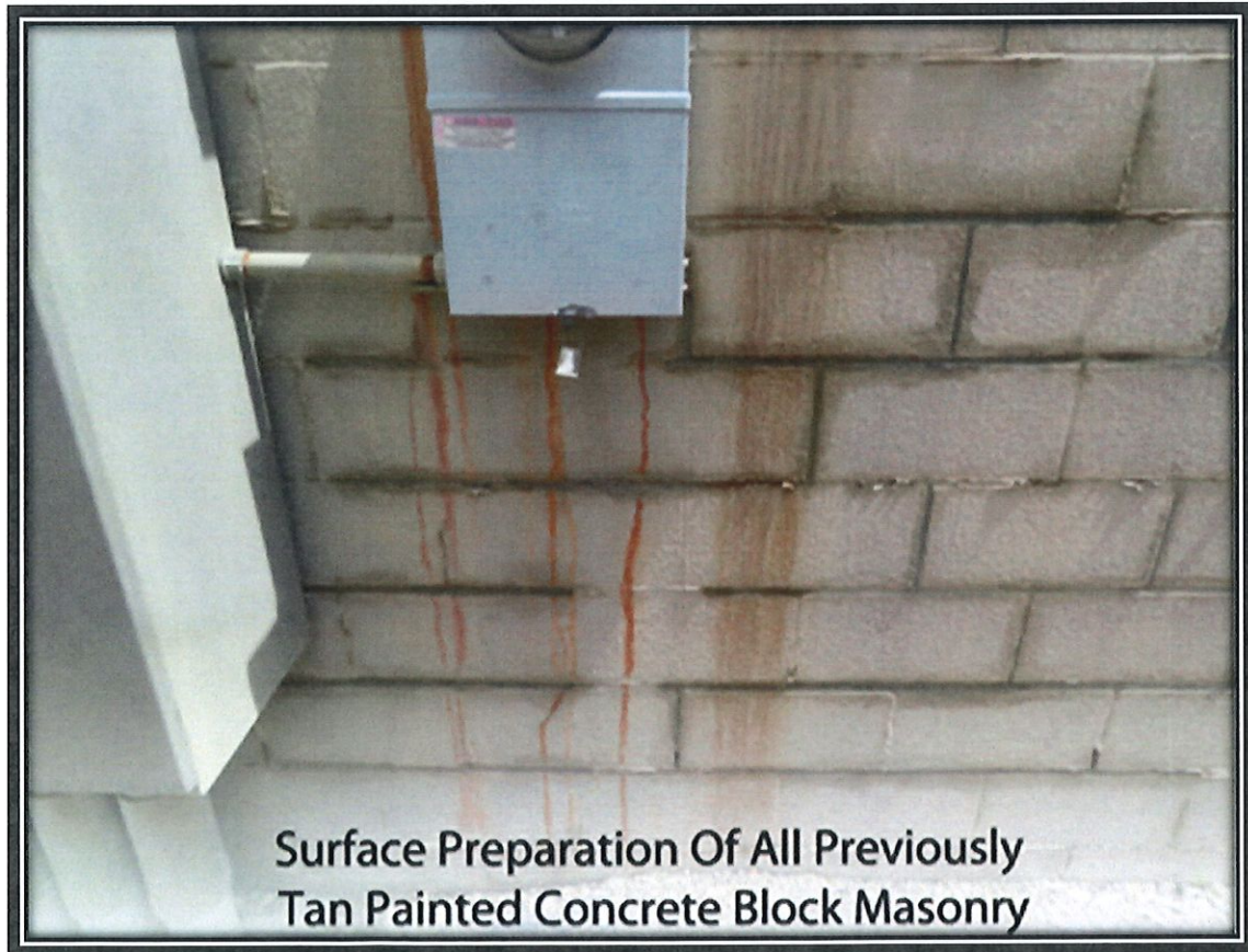
Surface Preparation Of All Previously Tan Painted Concrete Block Masonry
