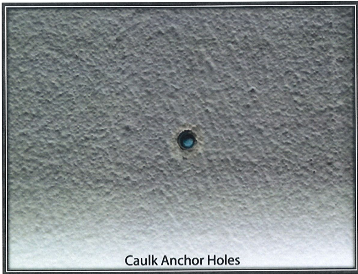
Caulk Anchor Holes
