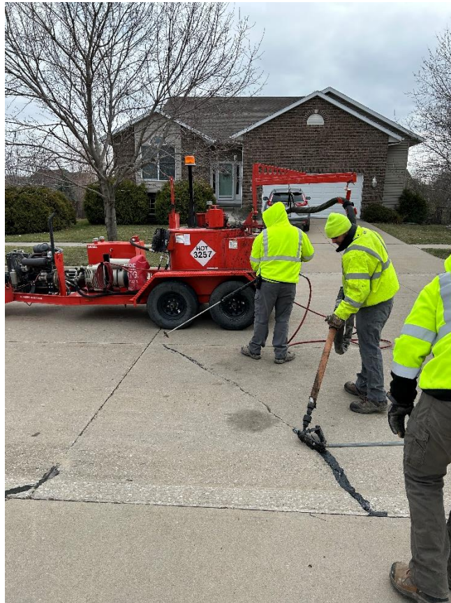
Crews performing crack sealing of streets to increase life of structures
