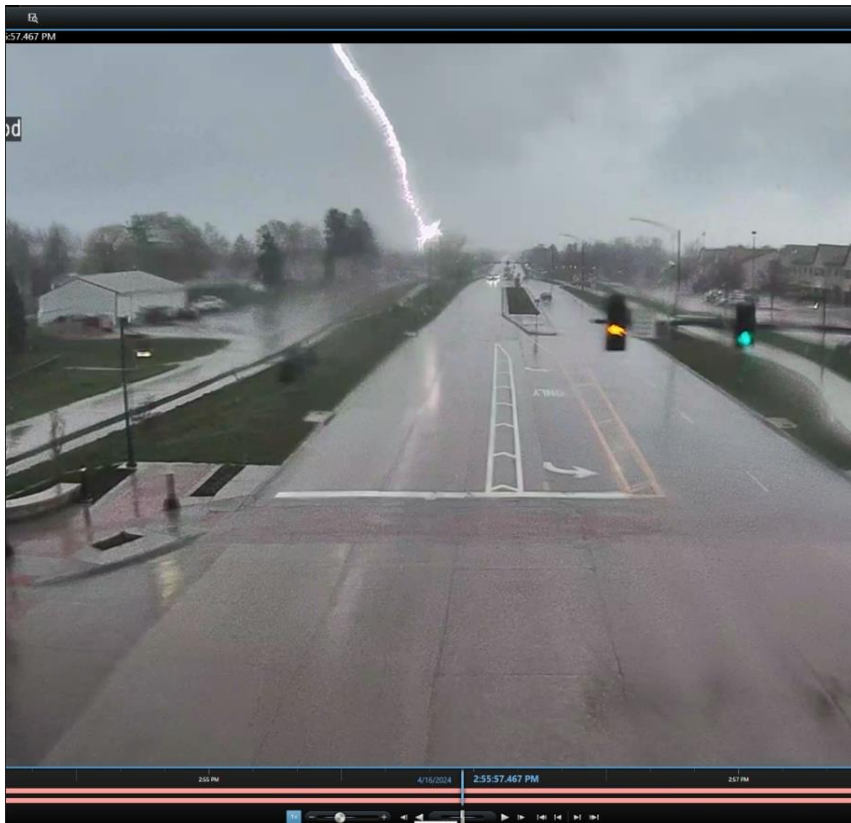
Lightning damage on Ranshaw Way striking streetlight
