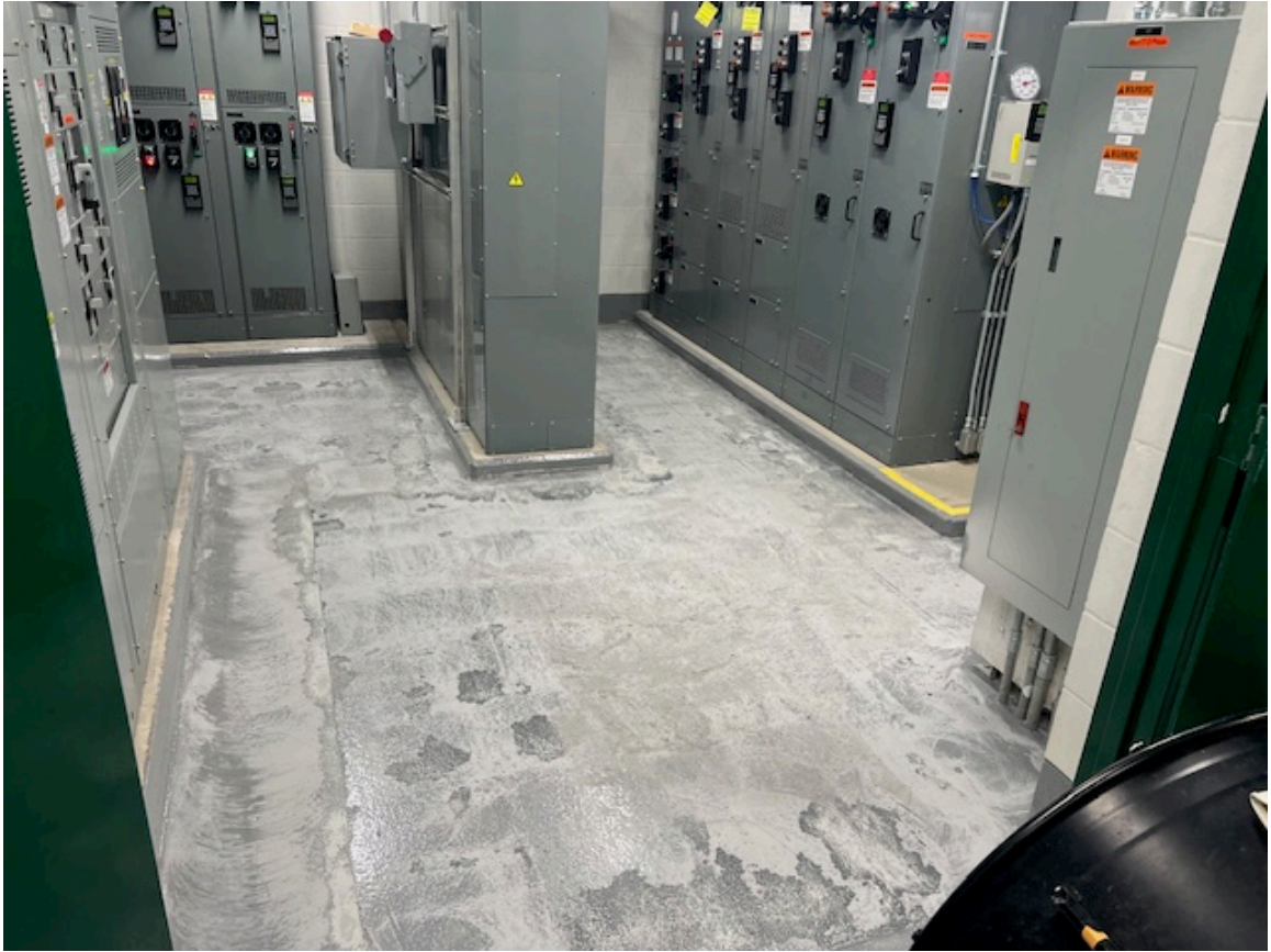
MBR Floor Coating Removal and Surface Prep
