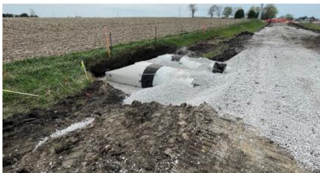
West Penn St road project storm pipe installed
