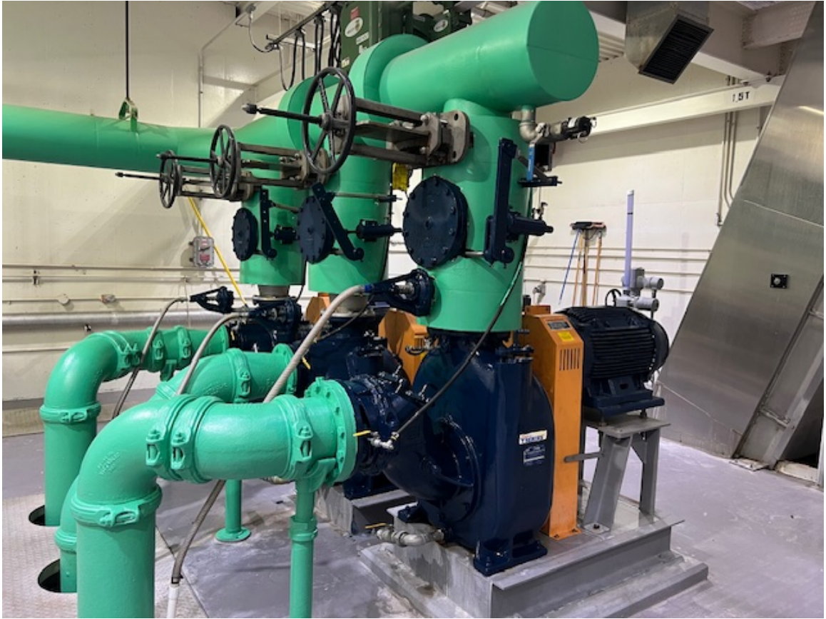
Main Lift Pumps and Piping Repainted
