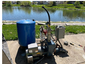
Irrigation pump replacement at Liberty Centre Pond.
