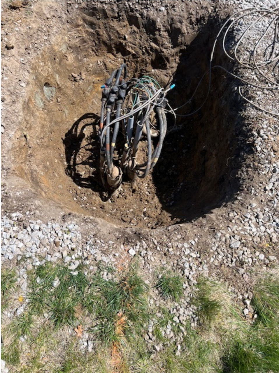
EQ Handhole removed and dug out
