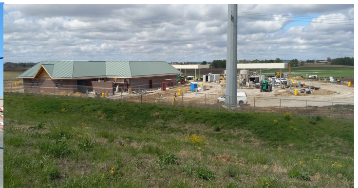
Kwik Star building shell and canopies installation completed
