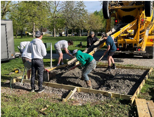
Liberty High School Construction Tech students pouring the concrete foundation pad for the new shed at the Community Gardens site next to Penn Meadows Park.
