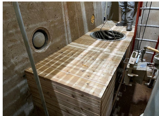
Filtration structure replacement at the indoor pool mechanical room.
