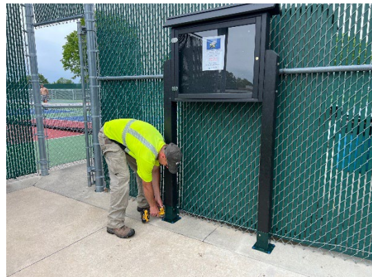
Info kiosk installed at the Tennis/Pickleball courts.
