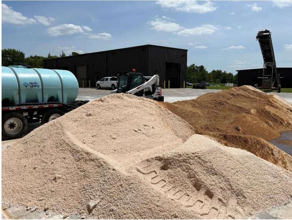
Mixing AG64 additive to road salt to improve ice/snow melting characteristics
