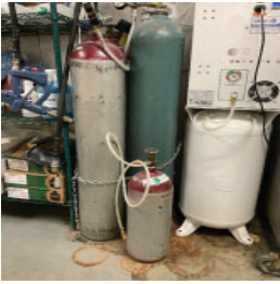
Not all cylinders secured
