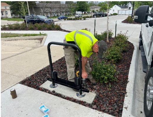
Boot scraper installed at City Hall.
