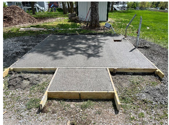
Liberty High School Construction Tech students pouring the concrete foundation pad for the new shed at the Community Gardens site next to Penn Meadows Park.
