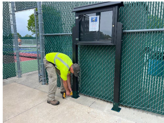
Info kiosk installed at the Tennis/Pickleball courts.
