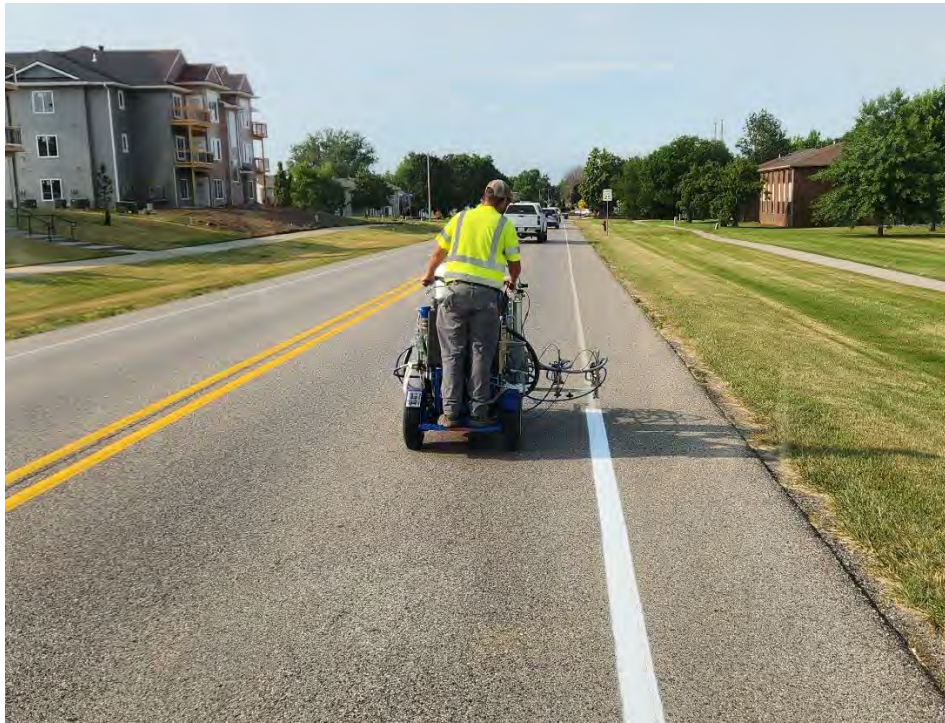
Staff painting streets with newly purchased equipment
