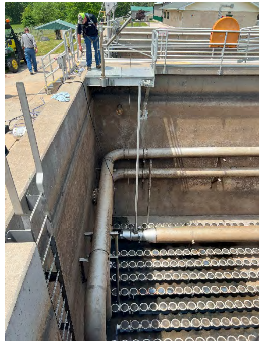
New Anoxic Return Pump Installation
