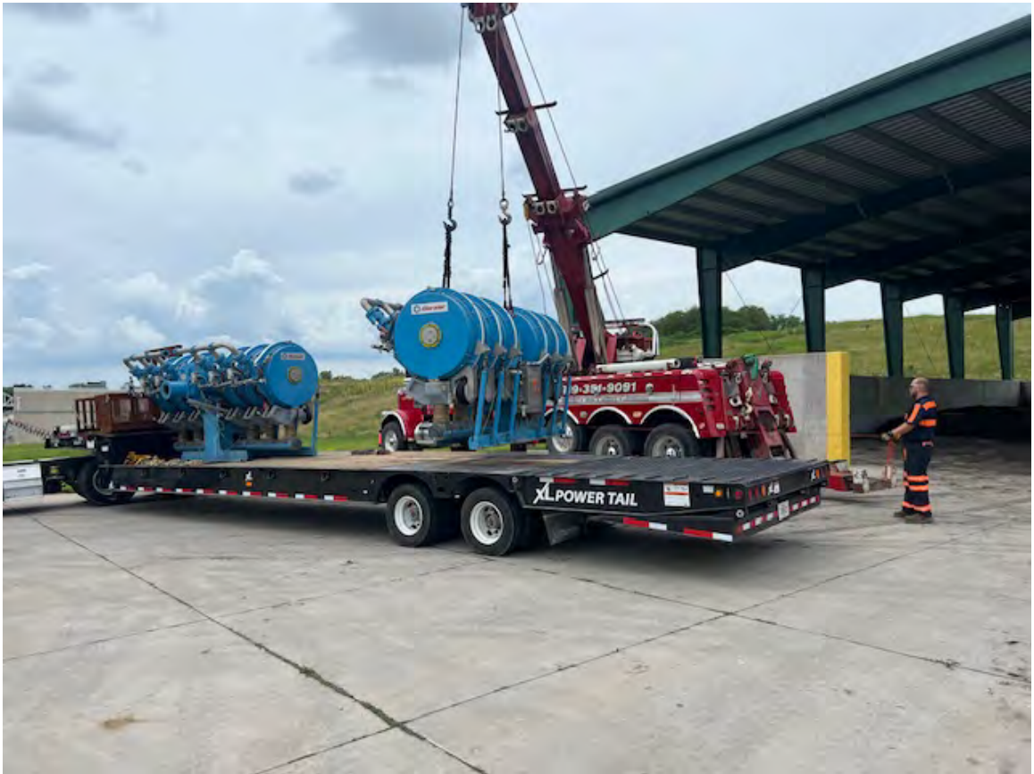
Unloading equipment at North Liberty WPCP
