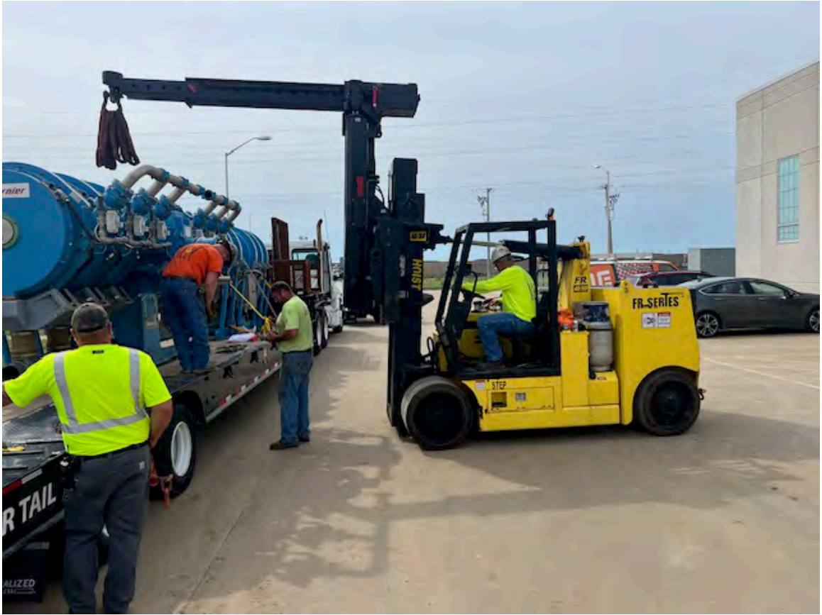
Loading used dewatering equipment purchased from City of Clinton
