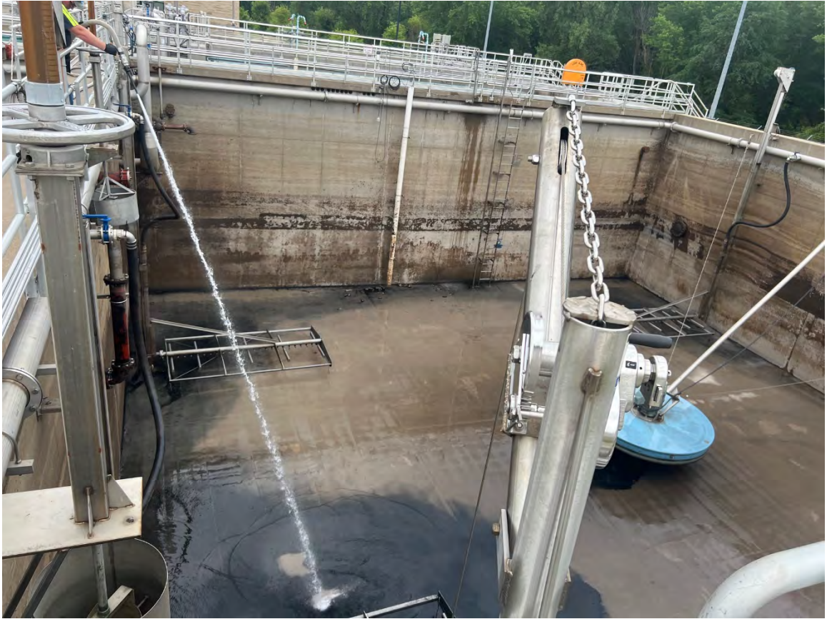
Digester cleaning and sediment pumped prior to tank inspection.
