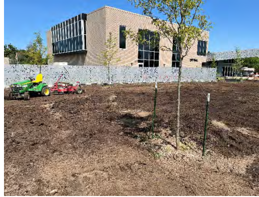
City Hall with staff adding compost and grading prior to sod installation.
