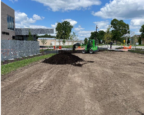
City Hall with staff adding compost and grading prior to sod installation.
