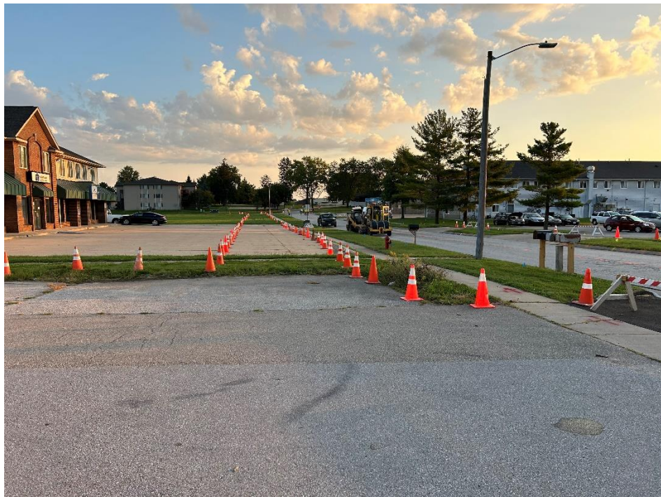
Sugar Creek temporary access
