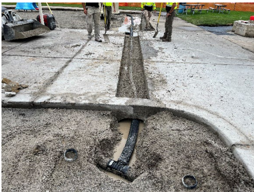
Park staff installing new ADS drainage tile and compacted rock base Penn Meadows Park.
