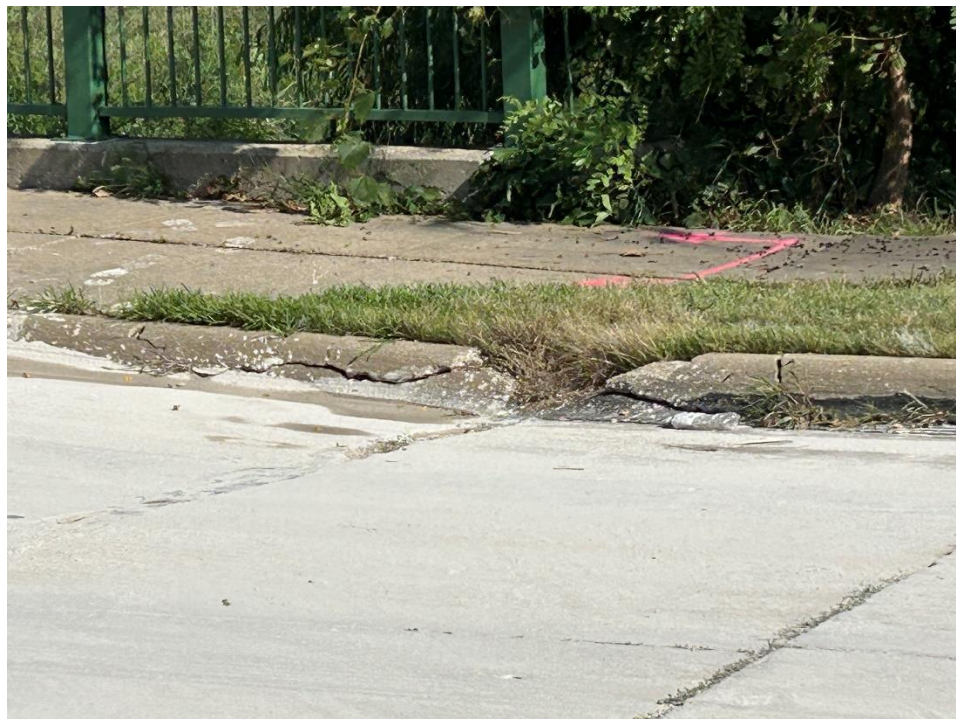
Rachael St repairs
