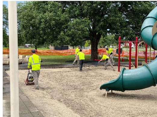
Park staff installing new ADS drainage tile and compacted rock base Penn Meadows Park.
