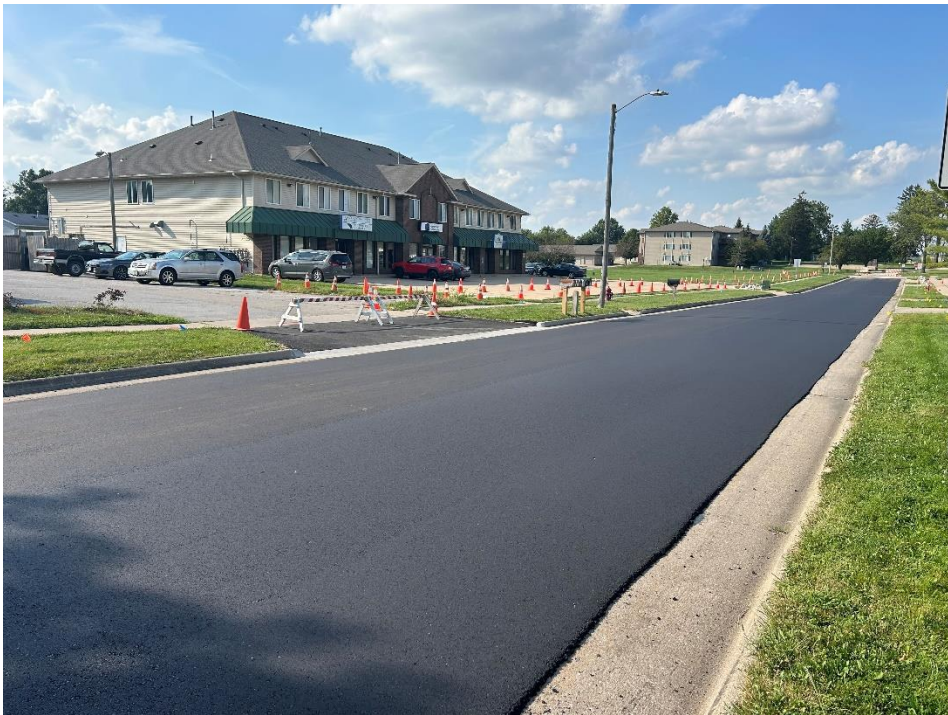
Sugar Creek Ln repairs
