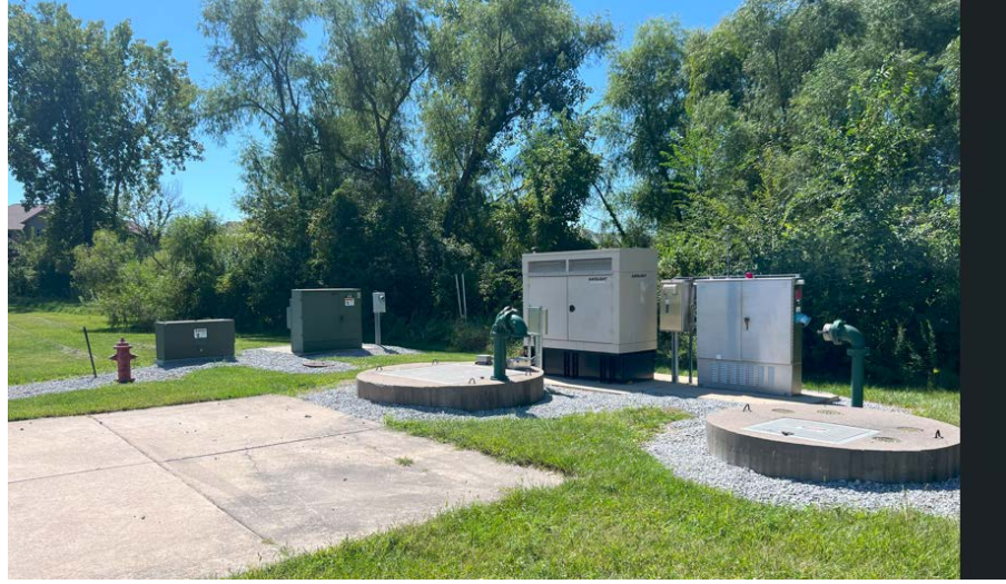
New rock around lift station equipment.
