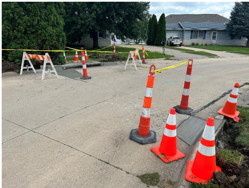
Prairie Ridge Ct repairs
