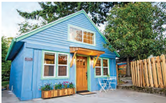
▲ Renting out this 350-square-foot garage-conversion ADU in Portland, Oregon, helps the property owner, who lives in the lot’s primary residence, pay her home mortgage.
