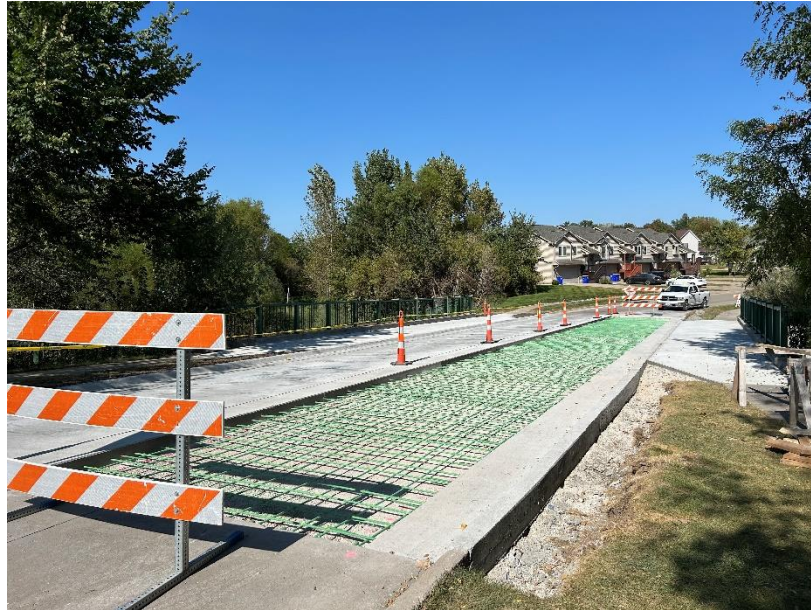
Reinforced steel matting embedded in road before the pour
