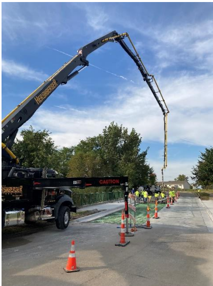
Reinforced steel matting embedded in road before the pour
