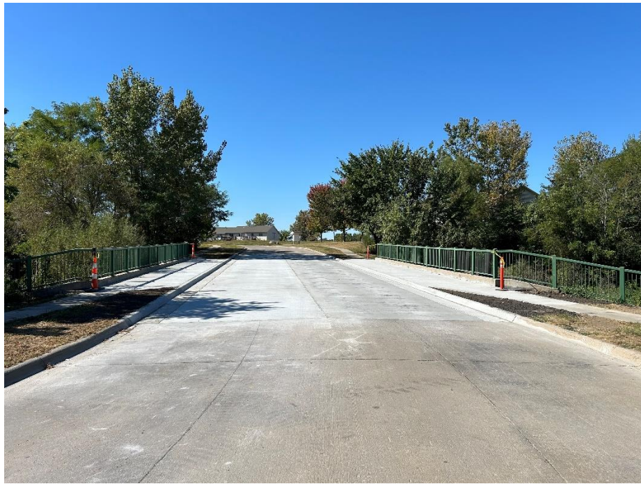
Completed Rachael St road project
