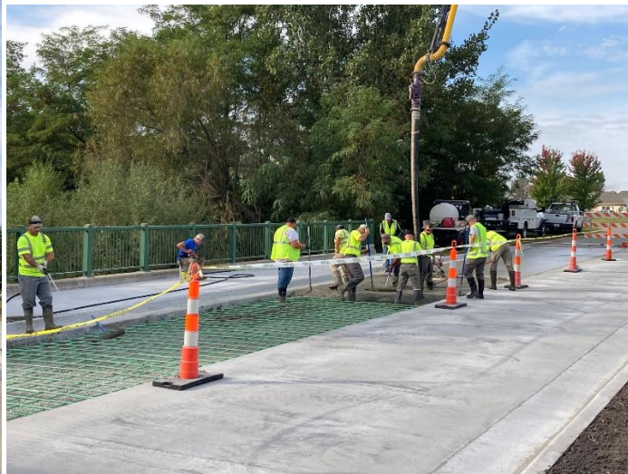
Staff pouring the south half of the road
