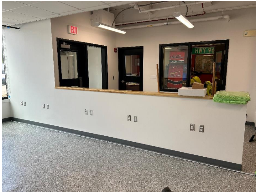
New office area in Street Department building project
