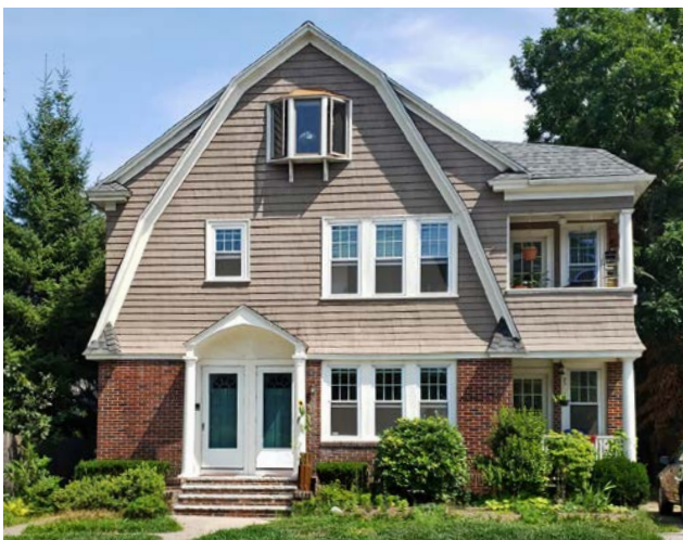
▲ Providence, Rhode Island, has many homes that were built as or long-ago converted into multidwelling units. (Notice the two front doors.) A homeowner can live in one apartment while renting out the other.
