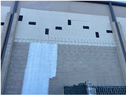
Rec Center tuckpointing and painting project underway.
