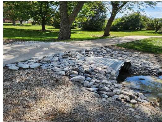
Riprap stone placed at West Lakes and Beaver Kreek Park for erosion control.
