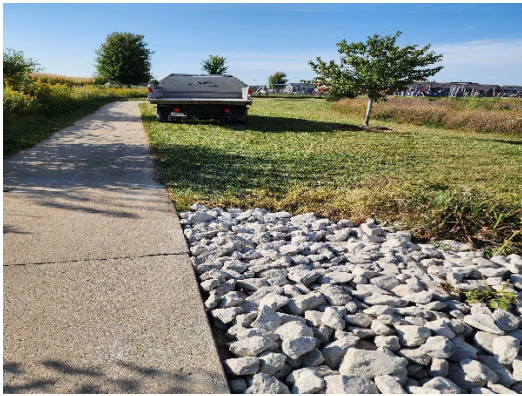
Riprap stone placed at West Lakes and Beaver Kreek Park for erosion control.
