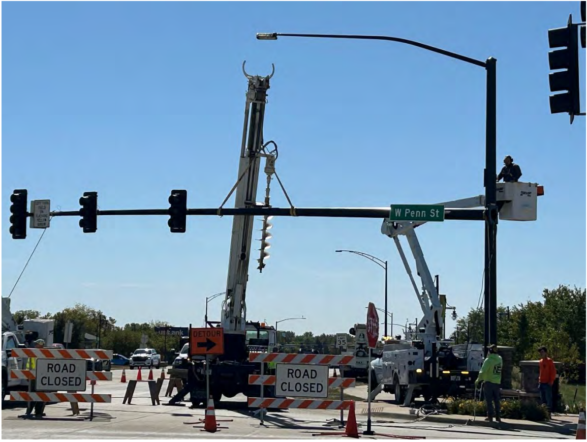
Ranshaw Way and W Penn St traffic signal removal and replacement
