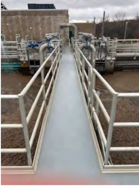
Completed Walkway with Epoxy Coating
