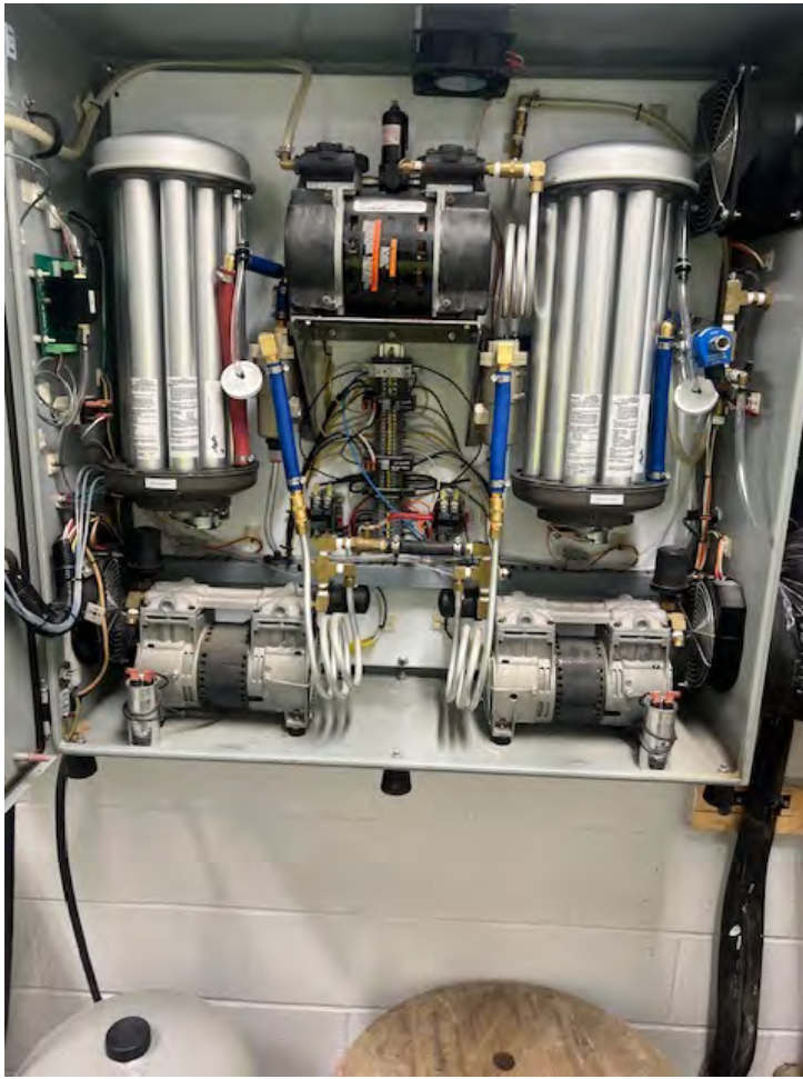
Rebuilt Oxygen Generator
