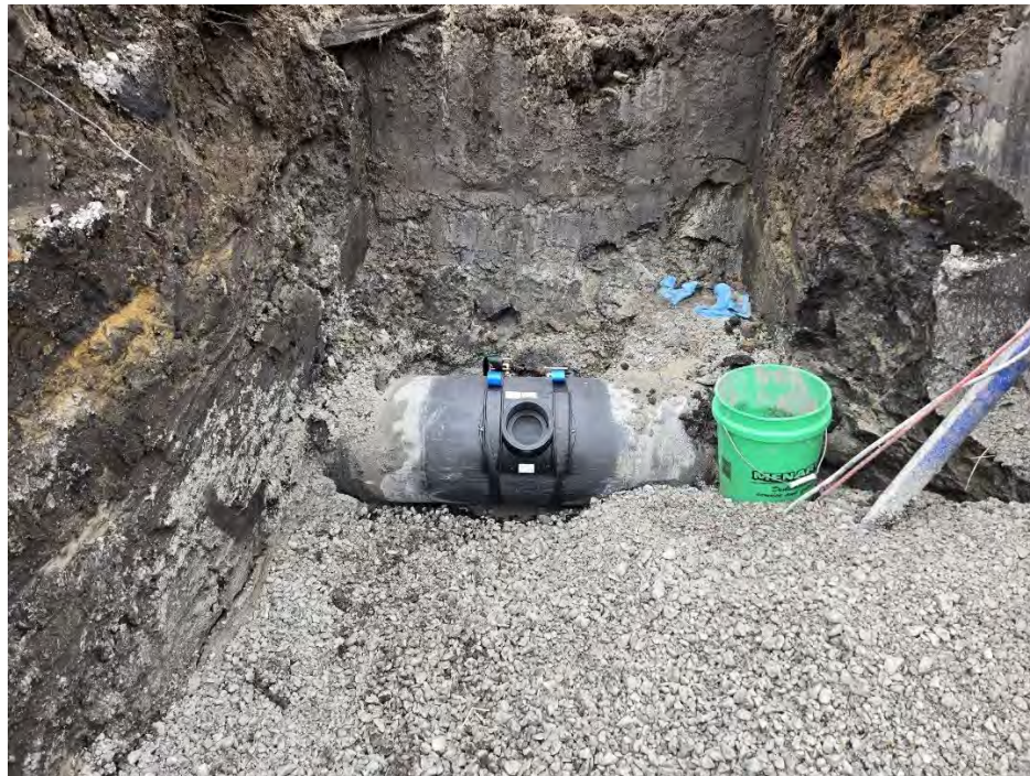
Food Pantry sewer service tap by electrofusion
