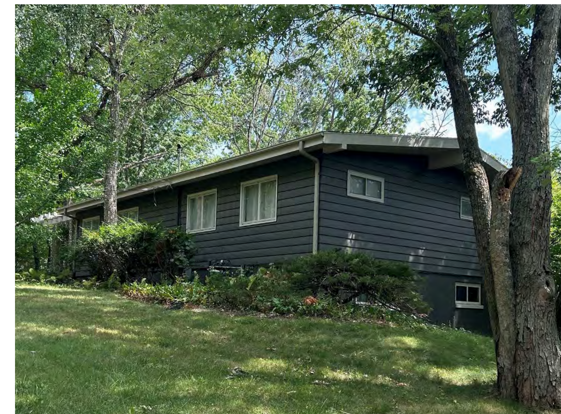
▲ LOWER LEVEL ADU Can be created through the conversion of a home's existing basement (provided that height and safety conditions are met), during construction of the house, or as part of a foundation replacement.
