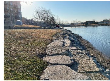
City Staff added rip rap rock at Liberty Centre. Completion of the outcropping repair project.
