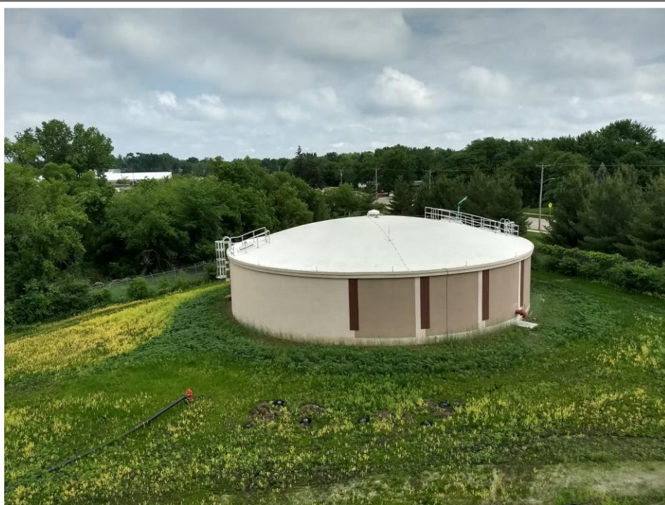
Figure 3.03-3 Ground Storage Reservoir
