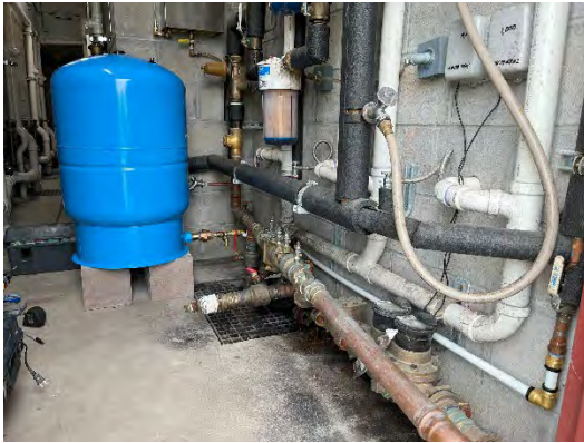
New pressure tank at Penn Meadows restroom facility.
